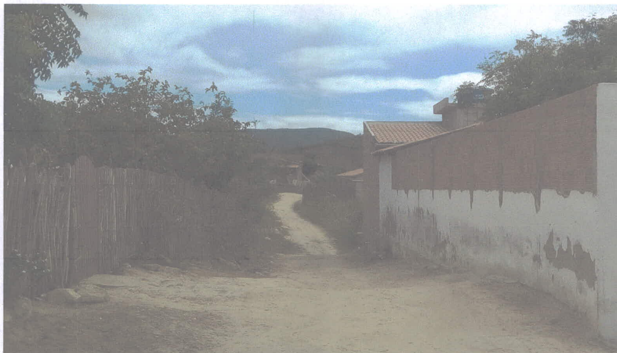
DIST. DE BANDEIRA – RUA SDO (INICIO) (E=447480.233 ; N=9493375.107)
